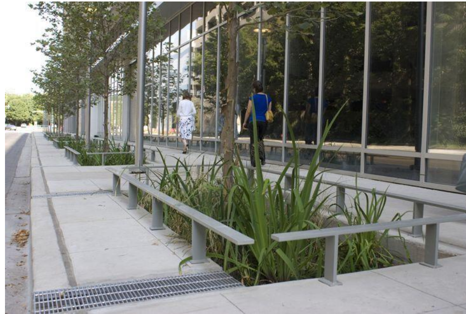
Foto: Stormwater infiltration planters at the Rush University Medical Center in Chicago (City of Chicago)
